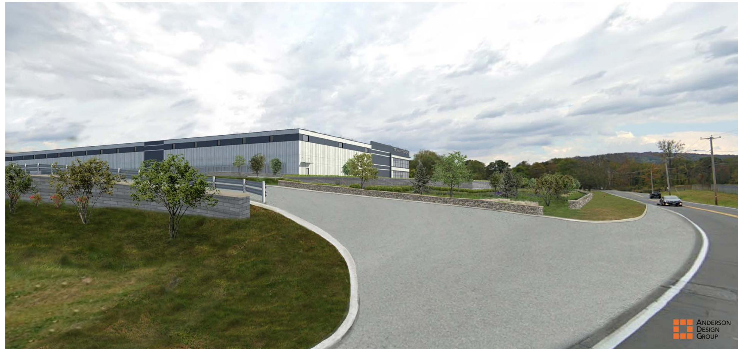
② VIEW FROM OLD LITTLE BRITAIN ROAD (LANDSCAPING AT YEAR 1) VANTAGE POINT 1
